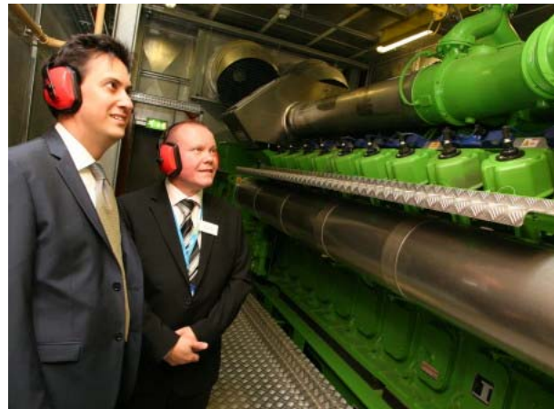
Ed Miliband with the hospital's head of engineering David Porter at the St Thomas' Jenbacher J620 CHP engine.
