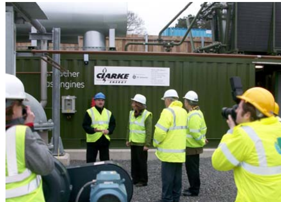
Clarke Energy Service Engineer, Glyn Wood, shows Jane Davidson, Minister for Environment, around the compound whilst under the glare of the local media.
